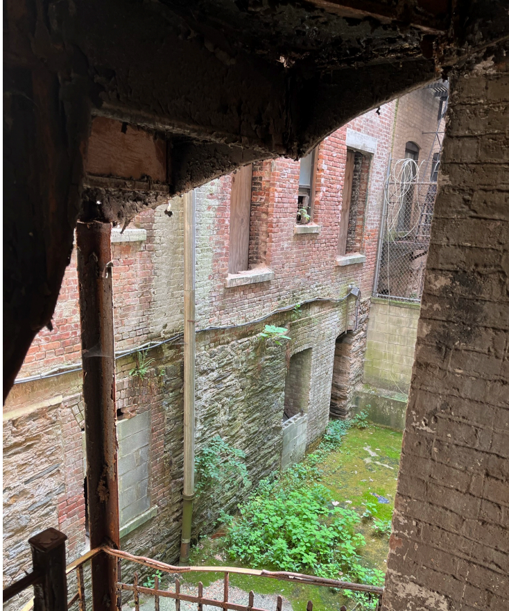
View of east courtyard from ground floor / exterior fire stairs
