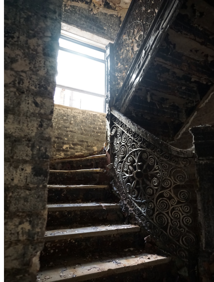
Existing interior stair – lobby level
